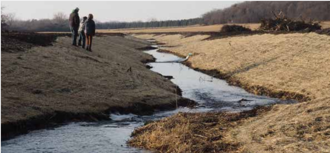
Post-project construction shows gentle sloping banks and stream curves designed to reduce flooding and erosion and improve water quality downstream in Green Lake.
